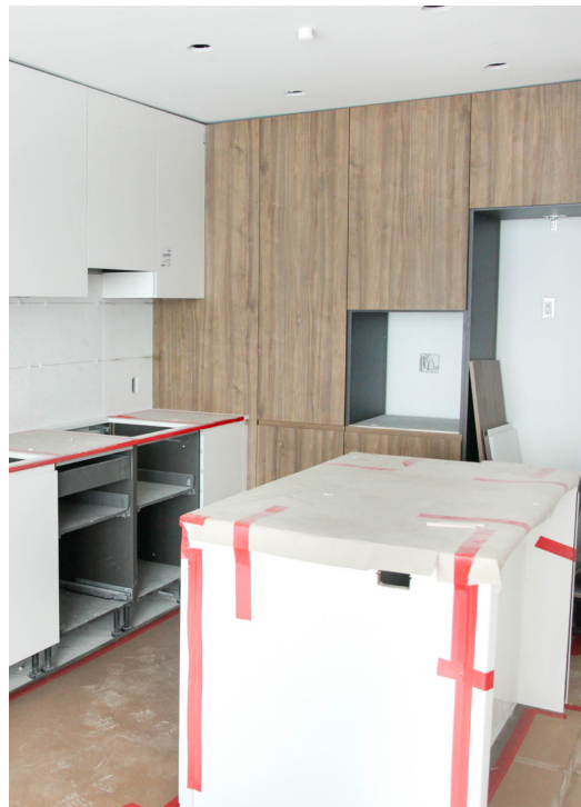
PROGRESS OF SUITES ON LEVEL 33 (FEBRUARY 2020)
