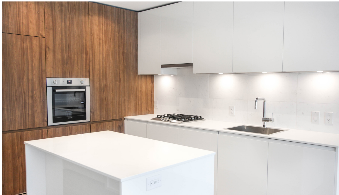
PROGRESS OF SUITES ON LEVEL 5 (FEBRUARY 2020)
