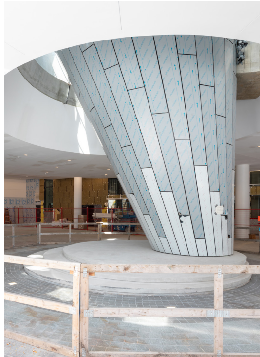
VIEW BELOW THE WATER FEATURE UNDER THE MAIN PLAZA (SEPTEMBER 2019)
