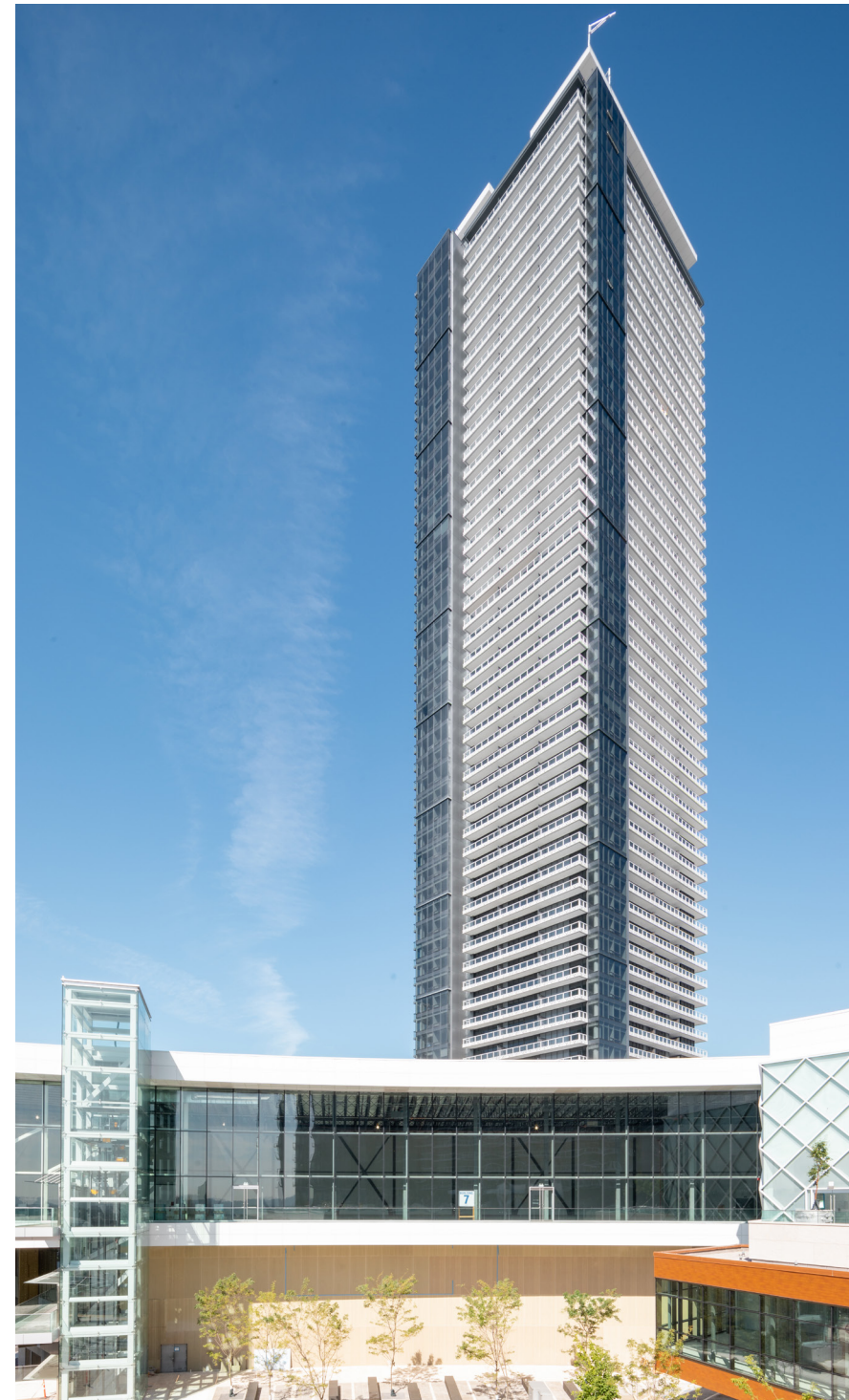
VIEW LOOKING TOWARDS CINEPLEX VIP AND TOWER ONE (SEPTEMBER 2019)
